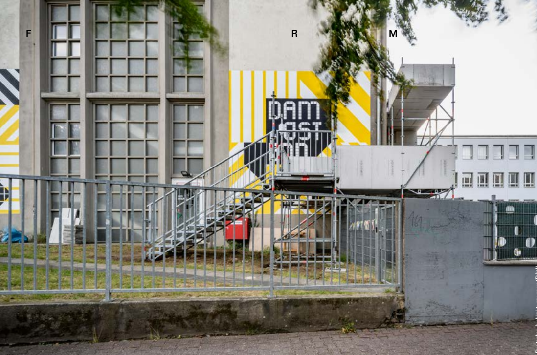
DAM Ostend in Frankfurt
