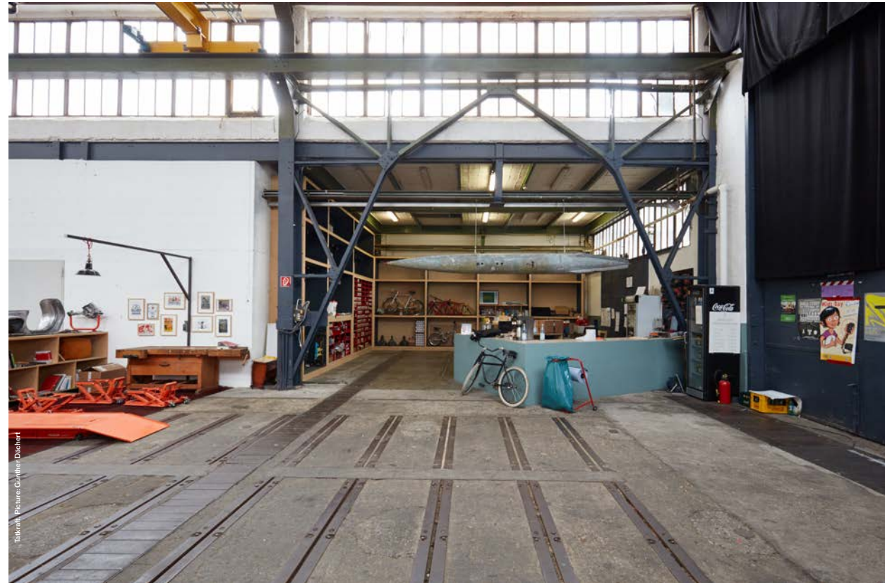
View into a former industrial space in Frankfurt-Seckbach
